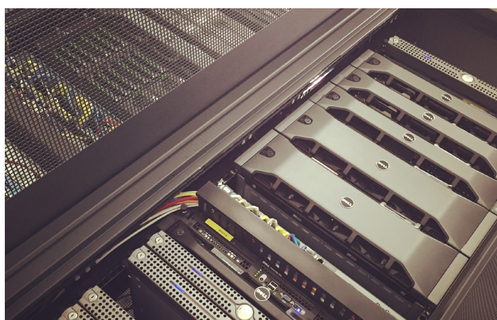
servers at a datacenter
